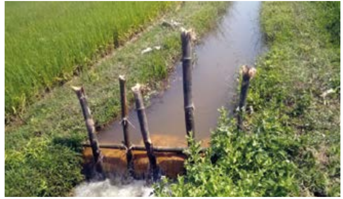
Figure 2.4: Controlling drainage flows from paddy farms to reduce discharge of drainage water and reusing it for irrigation. This improves irrigation efficiency, and reduces the demand for irrigation water from the rivers – and does not deplete the river flow and thus hinders saltwater intrusion, Vietnam. (Trinh Quoc Viet)
