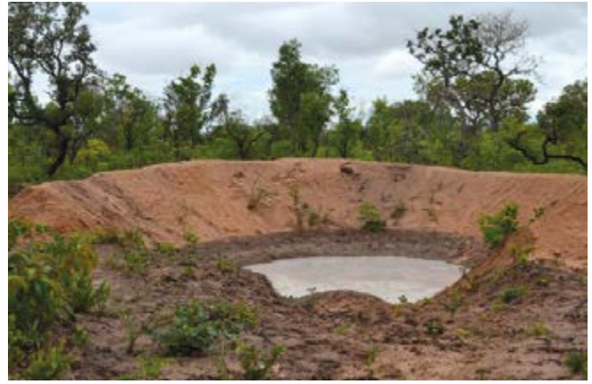
Figure 2.37: Barraginha – small pond for rainwater harvesting and control of sediment in the Bahian city of Cocos. ( http://cbhsaofrancisco.org.br/cbhsf/ )
