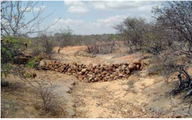
Figure 2.19: Dike (check dam) near to a Pankarará indigenous village shortly after construction (left), two years later with grass and trees (right), São Francisco River Basin, Brazil. (Pierson Barretto)
