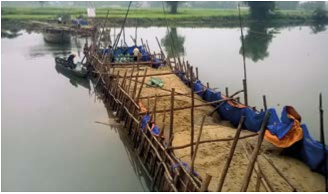
Figure 2.3: A temporary saltwater obstruction made of sand on the Vinh Dien River, Vietnam. These structures will be destroyed by the first floods of the wet season. (Trinh Quoc Viet)
