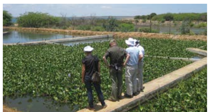
Figure 2.24: Green Liver System for treating aquaculture effluent, Brazil. (Johann Köppel)
